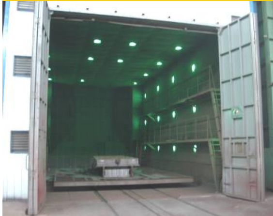
14m×10m×7m large size blasting shop
