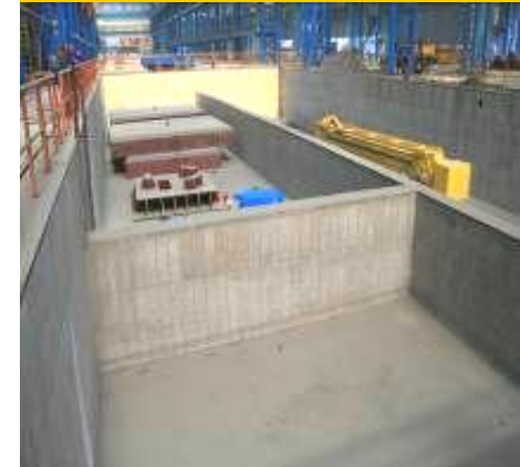
20m x 16m pouring pit 20m x 16m 浇注地坑
